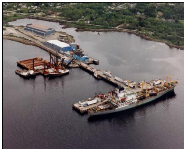
Figure 18.2 Aerial View of Ship-loading Facilities at Shelburne
