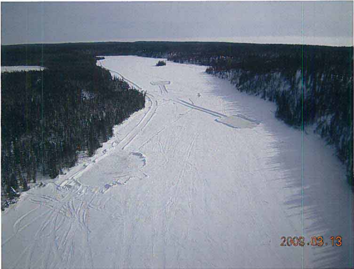
MV2007C0039 - Avalon Ventures Ltd. Two completed drill sites and two other ice pads being constructed.
