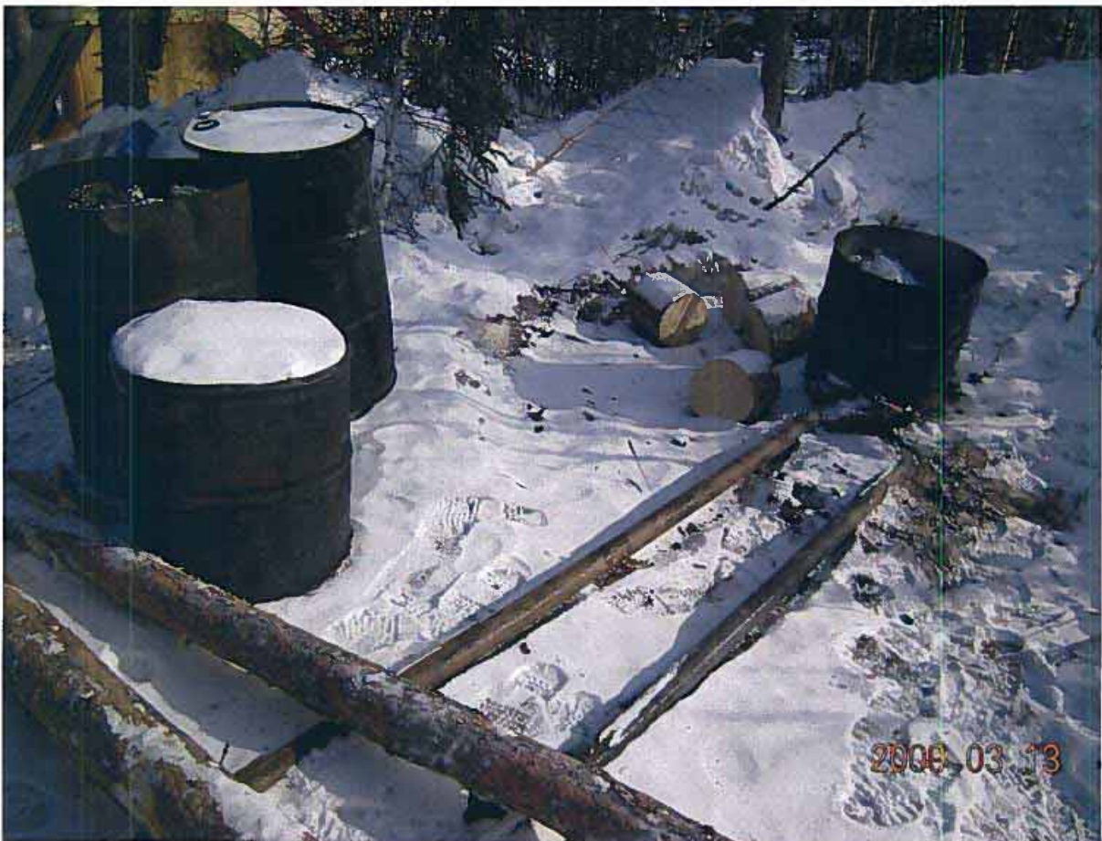
MV2007C0039 - Avalon Ventures Ltd. Barrels for the placement of hydrocarbon impacted snow/ice. Heated and absorbents used to mob up hydrocarbons.
